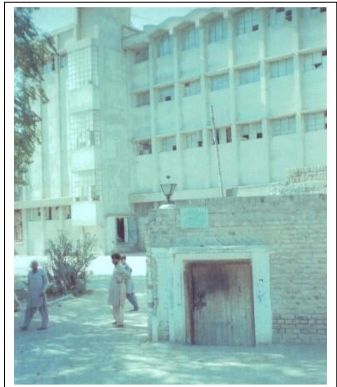
100 Ton / 24 hours grinding capacity Punjkora Flour Mill Timergarah Dir.
