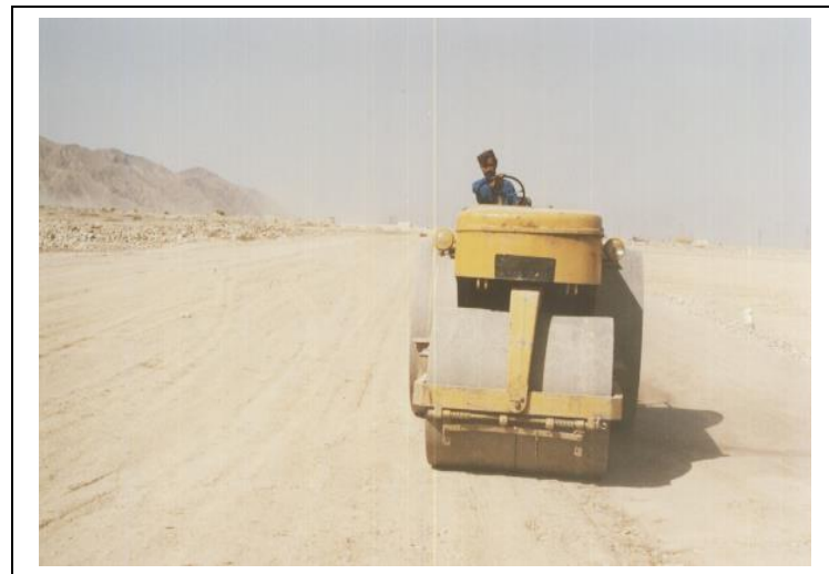
Preparing sub grade of internal roads
