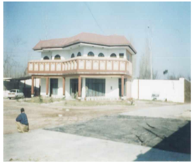
MD Office & Residence
