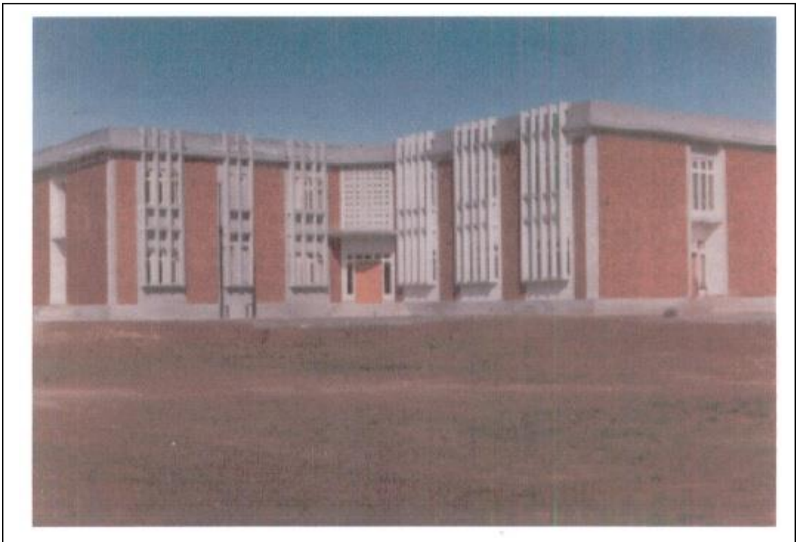
N-W.F.P., Forestry Pre-Investment Center Building
