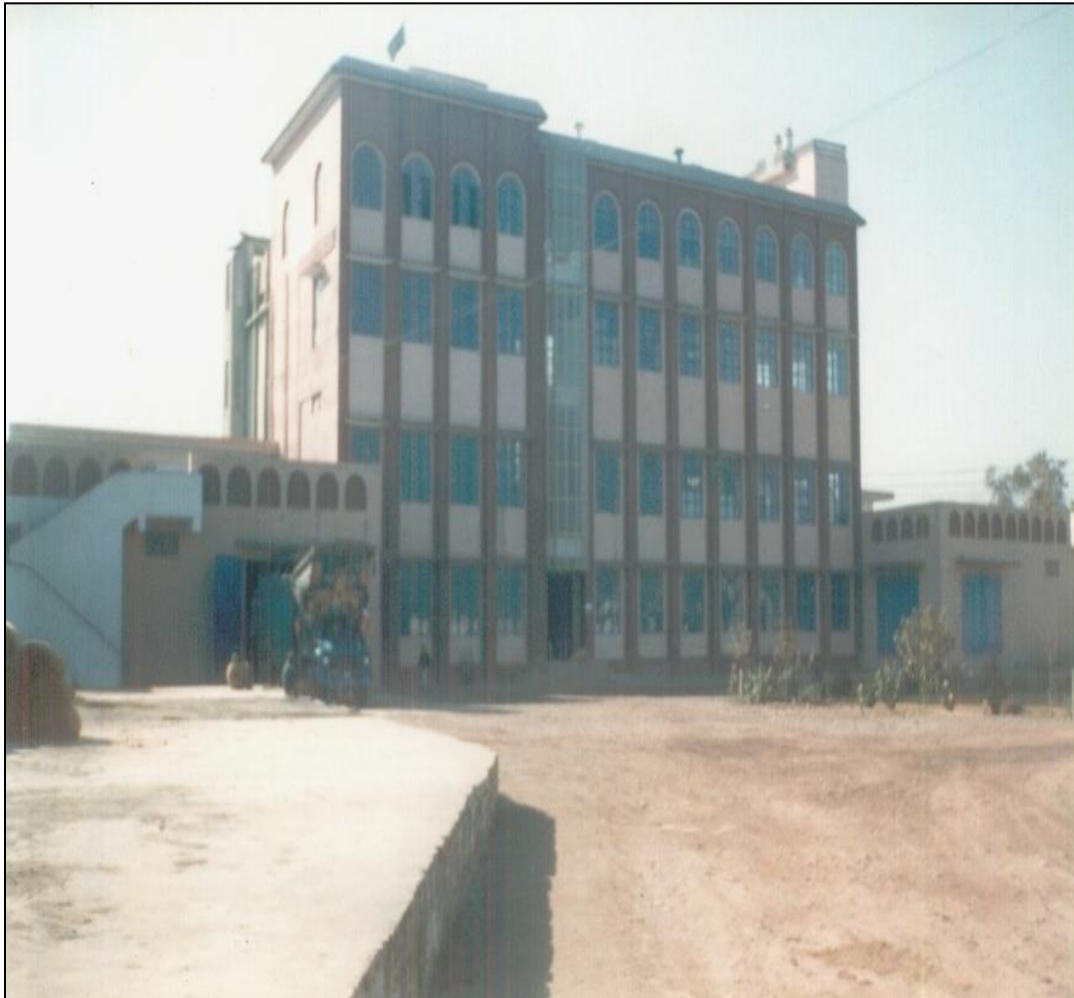
Zain Flour Mill Building Grinding Capacity 100 Ton / 24 hours
