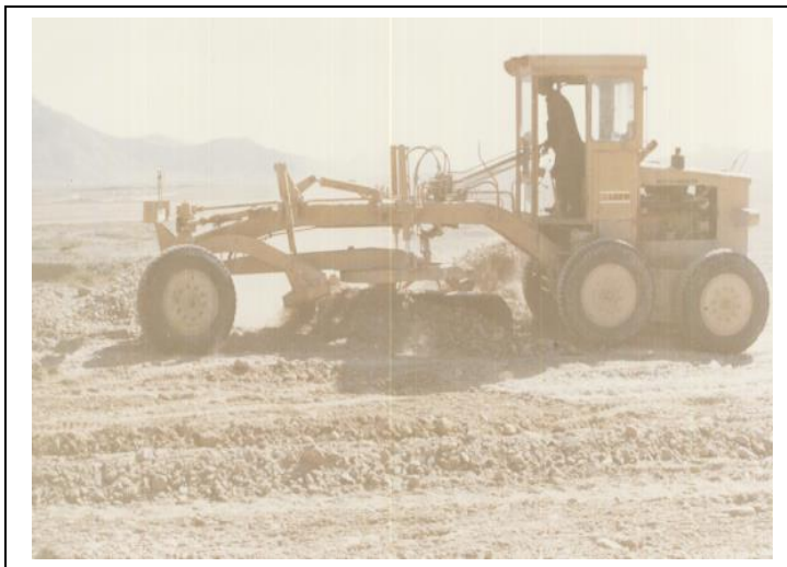
Grading leveling internal roads
